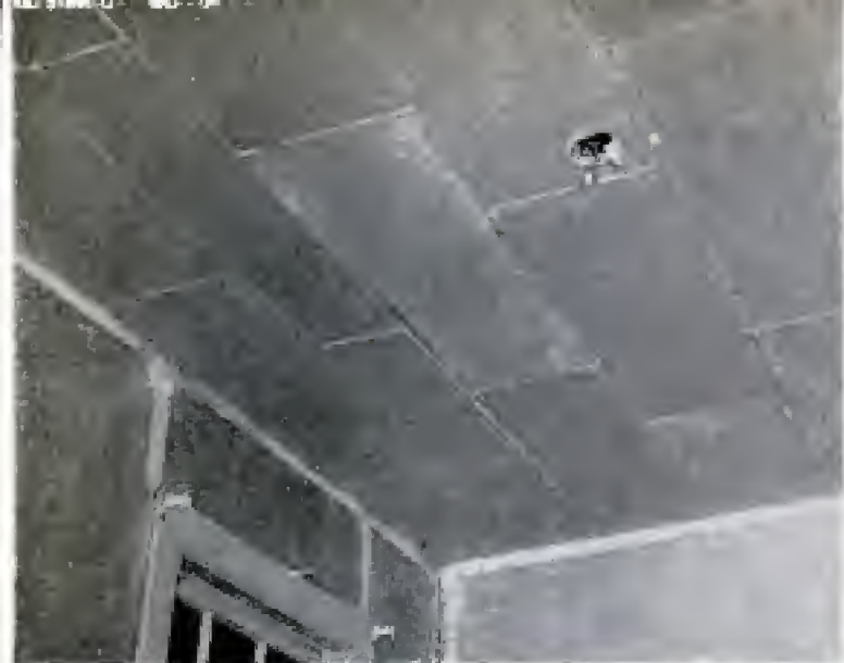
Original ceiling is completely covered with gypsum lath and ready for new plaster. Only a 1/2-in.-thick layer of plaster is required to cover the lath base
